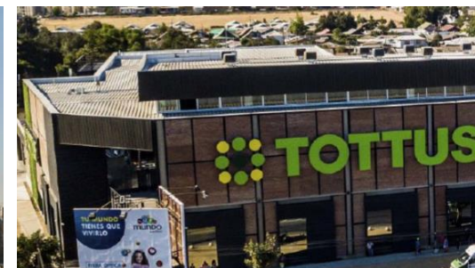
Power Center Curicó
